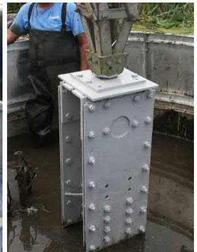
Repair of a severely deteriorated pile foundation on a 230 kV guyed mast transmission tower located in a protected wetland area.
