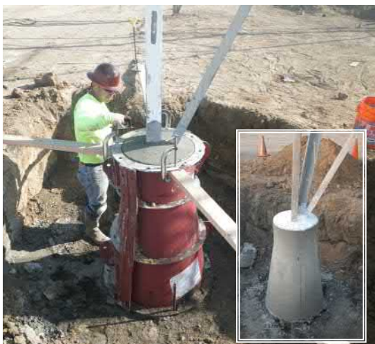
Reinforced concrete encasement of a severely corroded tower section.
