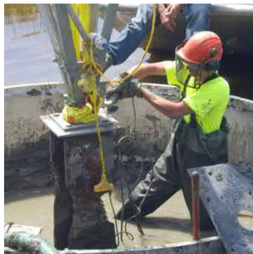
Repair of a severely deteriorated pile foundation on a 230 kV guyed mast transmission tower located in a protected wetland area.
